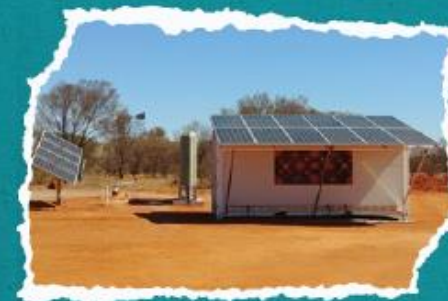
Project Gilghi, Australia (solar-powered water treatment plant)
